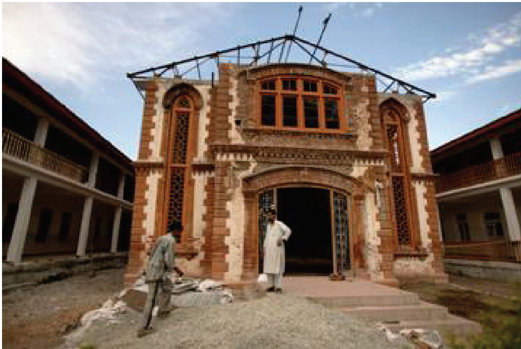
Laborers work on the reconstruction of the renowned Islamia High School in downtown Srinagar, August 2, 2005. The school suffered an arson attack in early 2005 by Pakistani-supported Islamist militants as a warning to the Kashmiri owner and religious leader of the school not to negotiate with the Indian Government over Kashmir's independence. © 2005 Robert Nickelsberg
